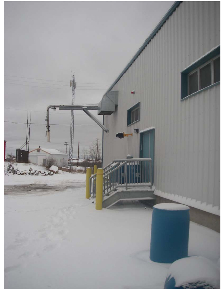
Rae Water Supply Facility
