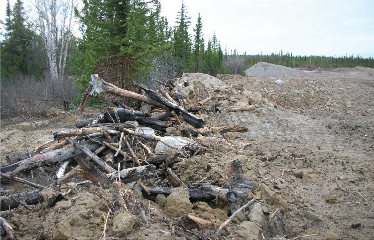
figure 20. Overburden and woody debris should not be mixed, and piles should be at least 5 m from standing timber.
