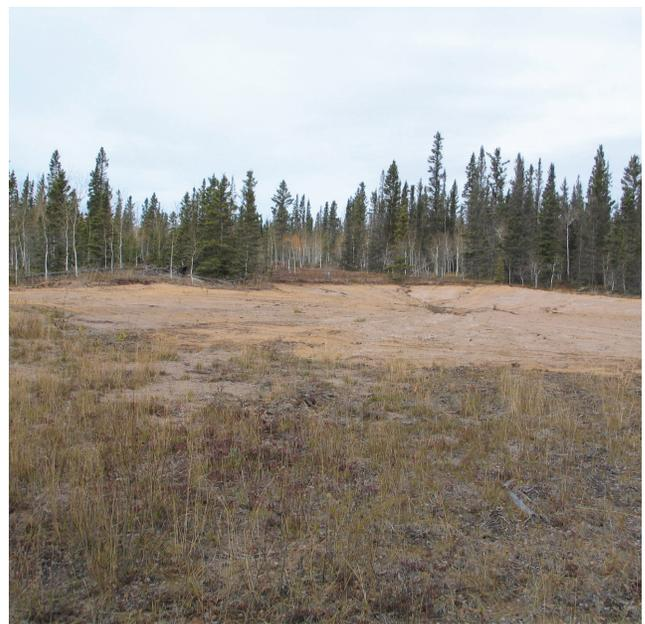
figure 23. This pit has been recontoured and left to revegetate naturally.
